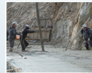
Large work area
