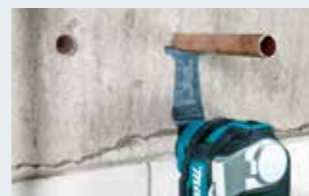
Copper pipe flush cutting
