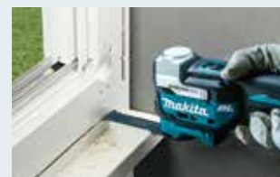
Removal of window frame
