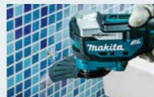
Routing joints on wall tiles
