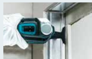
Door opening work
